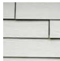
Gaps in Fiber Cement
